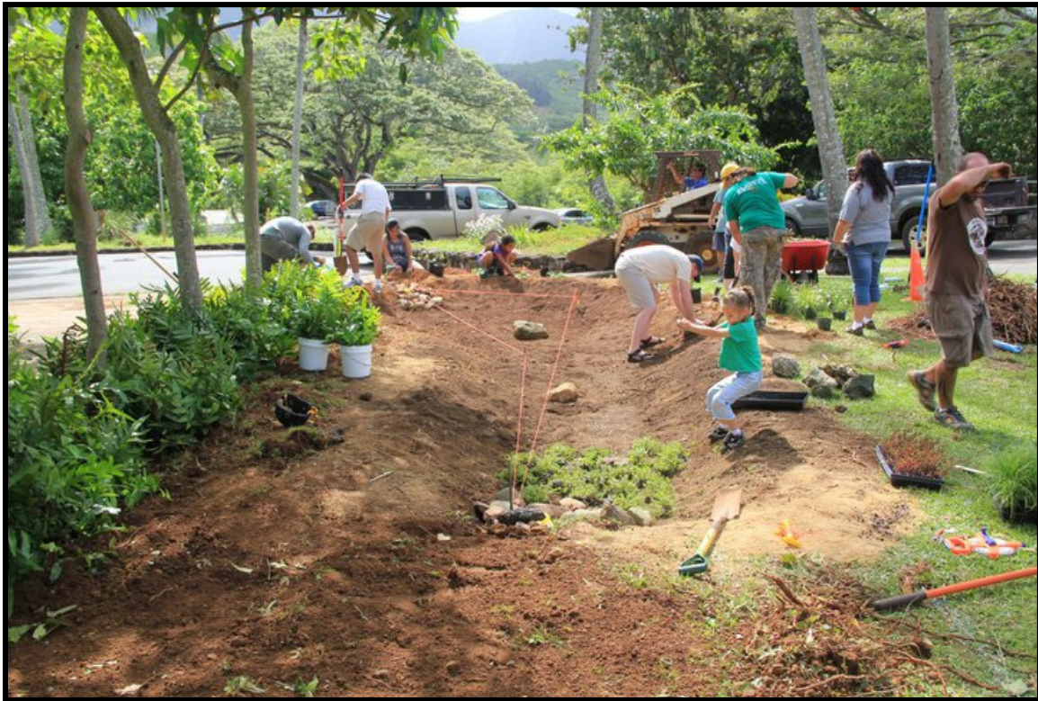
Figure 3 Rain Garden construction at He'eia State Park
