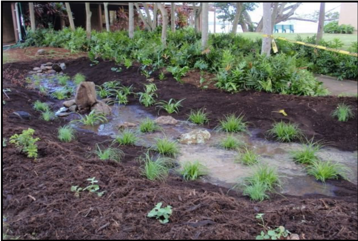
Figure 4 Completed Rain Garden at He'eia State Park
